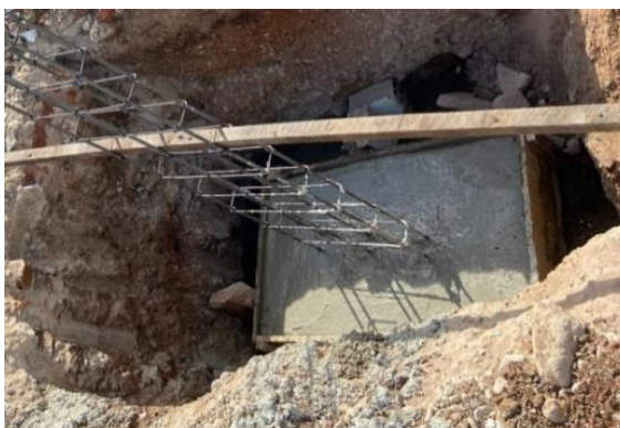
Figura 13 – Base concretada
